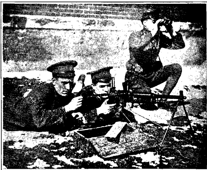
Thirty-five-pound, air-cooled machine gun, capable of firing 200 to 500 shots per minute
