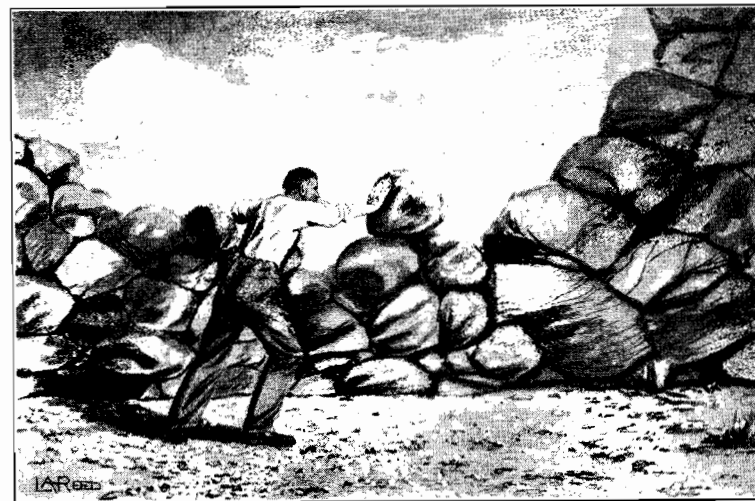
OPENING THE ROAD
