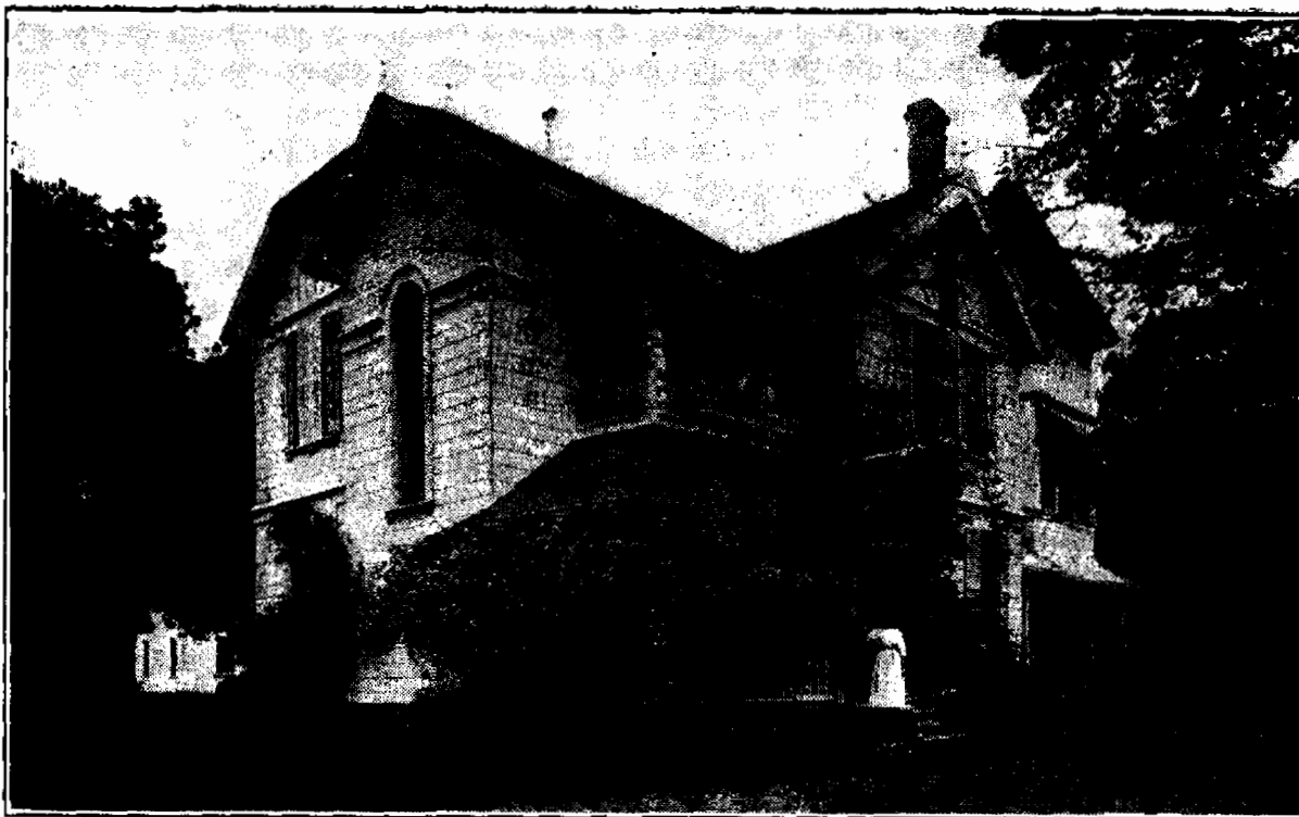
"ELMSHAVEN," HOME OF MRS. E. G. WHITE, NEAR ST. HELENA, CALIFORNIA
