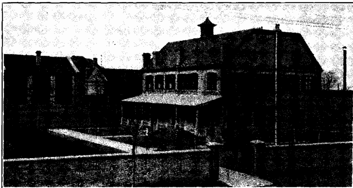
PUBLISHING HOUSE IN SHANGHAI, CHINA
