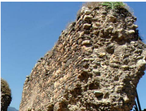
Section of old wall at Philadelphia
