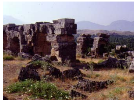
Section of Aqueduct of old Laodicea
